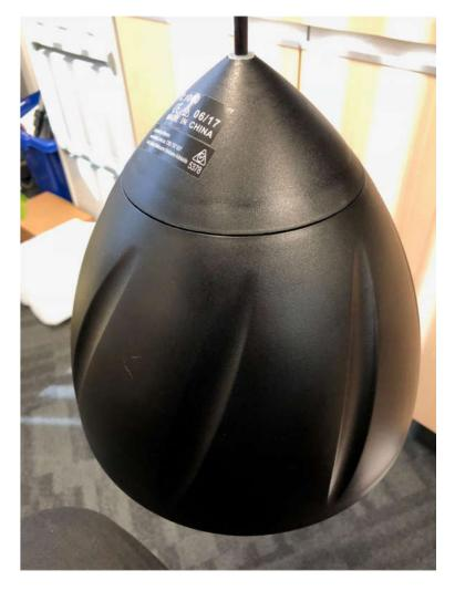
Thread cable through speaker cap& secure cap to speaker.
