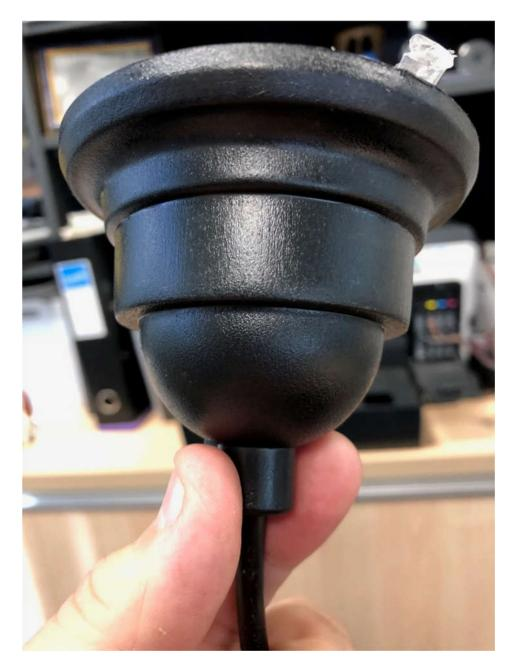
Push ceiling rose cover over the ceiling mount and tape in place using insulation tape.
