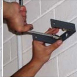
Step 5 Bolt or screw metal "U" bracket to wall.
