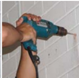
Step 2 Drill mounting holes.
