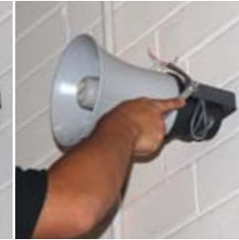
Step 7 Adjust horn angle and tighten bolts.
