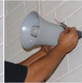
Step 6 Re-fix horn to metal "U" bracket.
