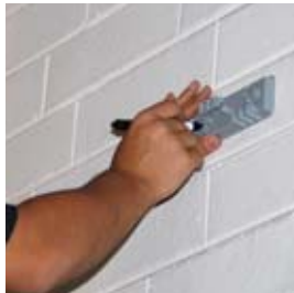
Step 1 Mark mounting holes for drilling.
