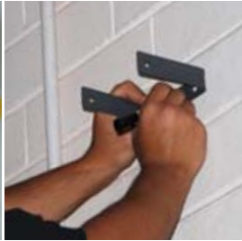
Step 2 Mark mounting holes for drilling.
